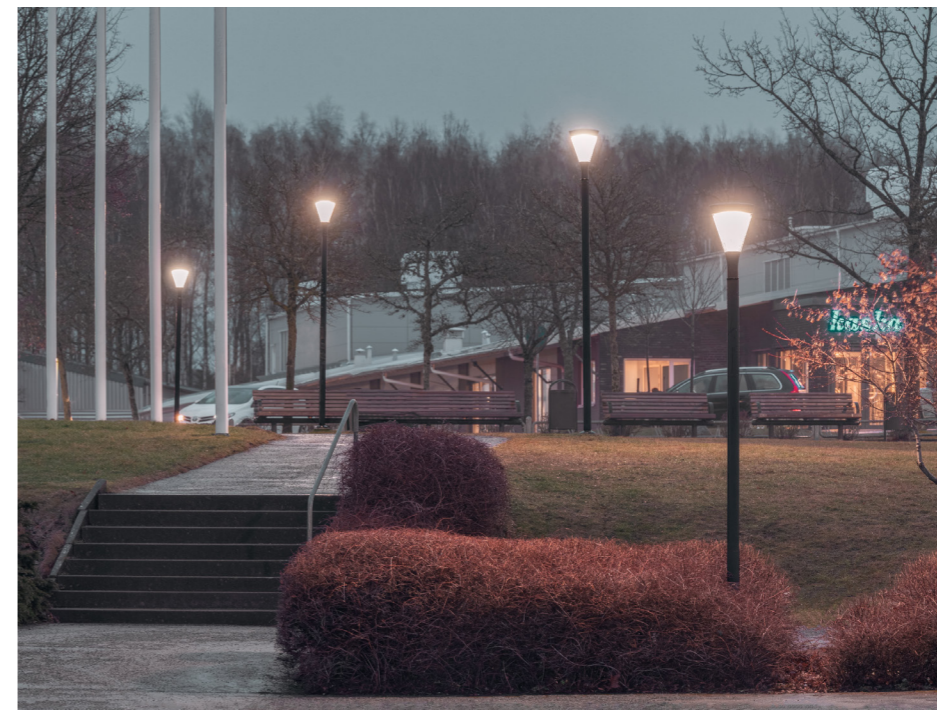
↳ Luscinia Post Top, Marks gymnasieskola, Kinna, Sweden
